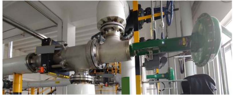
Figure 1 Prosonix Coaxial Jet cooker installation
